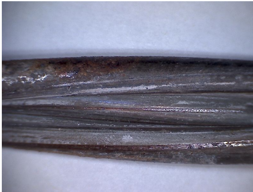
Figure 5-5 – Close up of a 7-wire strand as extracted from the beam after fatigue failure
