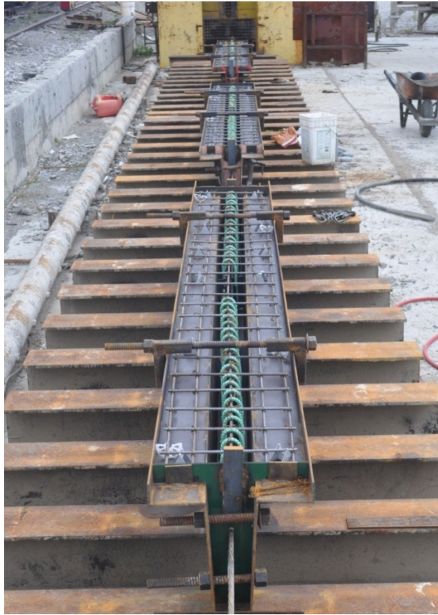
Figure 3-5 – Beam forms along the prestressing bed
