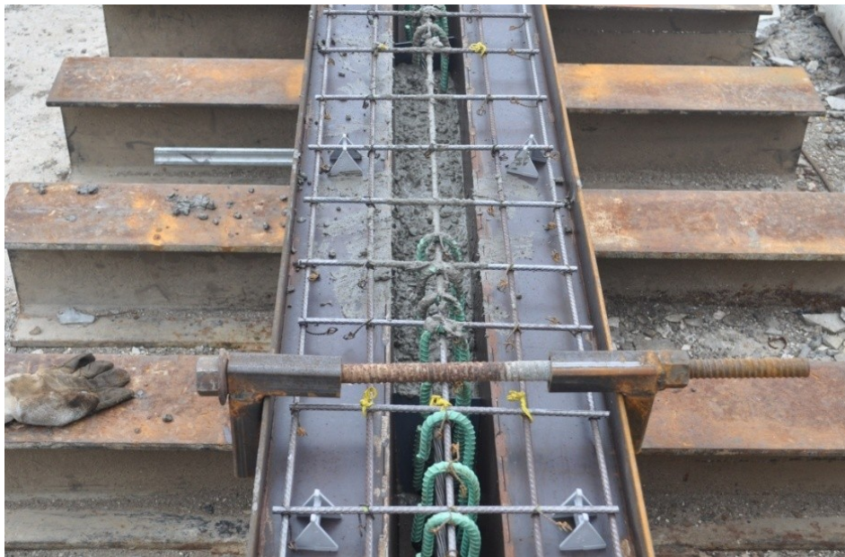
Figure 3-7 – Salted portion of the beam
