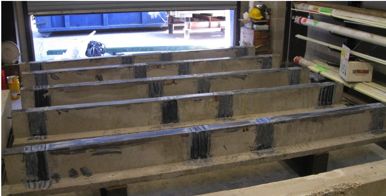
Figure 3-9 – Beams after application of CFRP sheet repair
