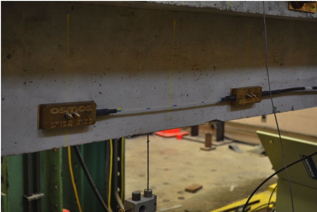
Figure 3-13 – OSMOS FOS across flexure zone for average strain readings at the level of the strand
