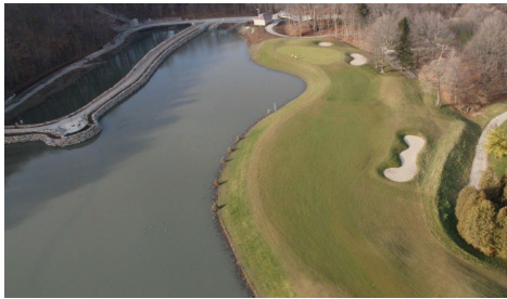
2.41 The site condition before the construction of Earl Bales Pond.
