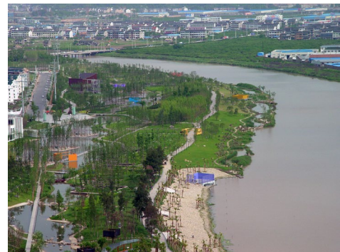
2.3 Bottom: The Yongning Park Project and layers of its landscape elements: it is composed of two layers: the natural matrix which is composed of wetland and natural vegetation designed for the natural processes of flooding and native habitats, and human matrix which is composed of a designed tree matrix, a path network, and a matrix of story boxes.
