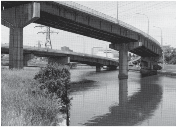
1.8 The urbanized channel of the Don.
