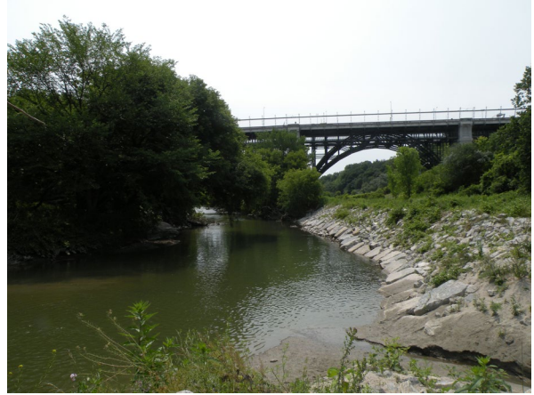
3.29 Existing condition of the river at location 2.
