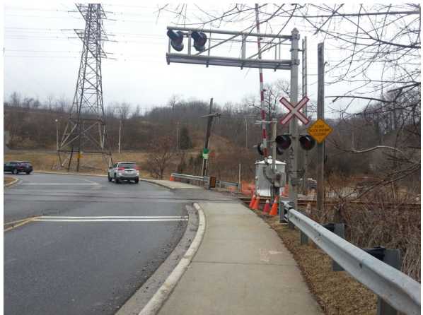
3.21 Pottery Road: sidewalk connects the parking to the Trailhead.
