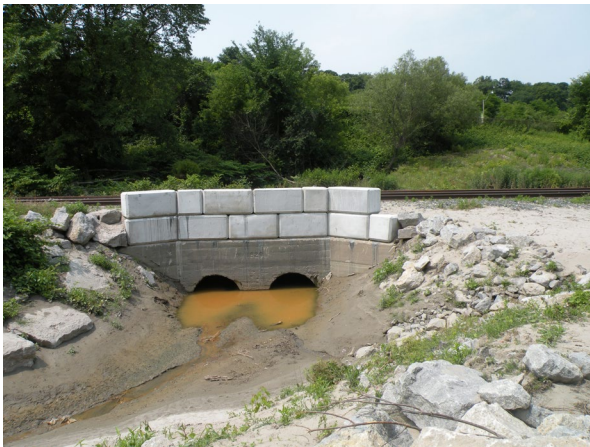
3.30 Existing outfalls at site location 2.
