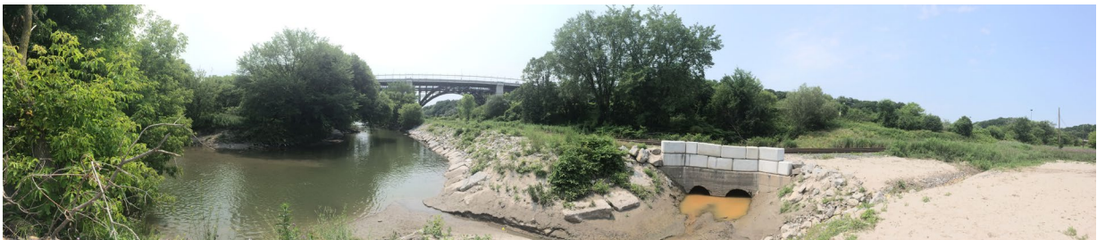
3.27 Panoramic view at location 2 showing the existing river's edge condition, outfalls, and the untreated water dumping into the Don River.
