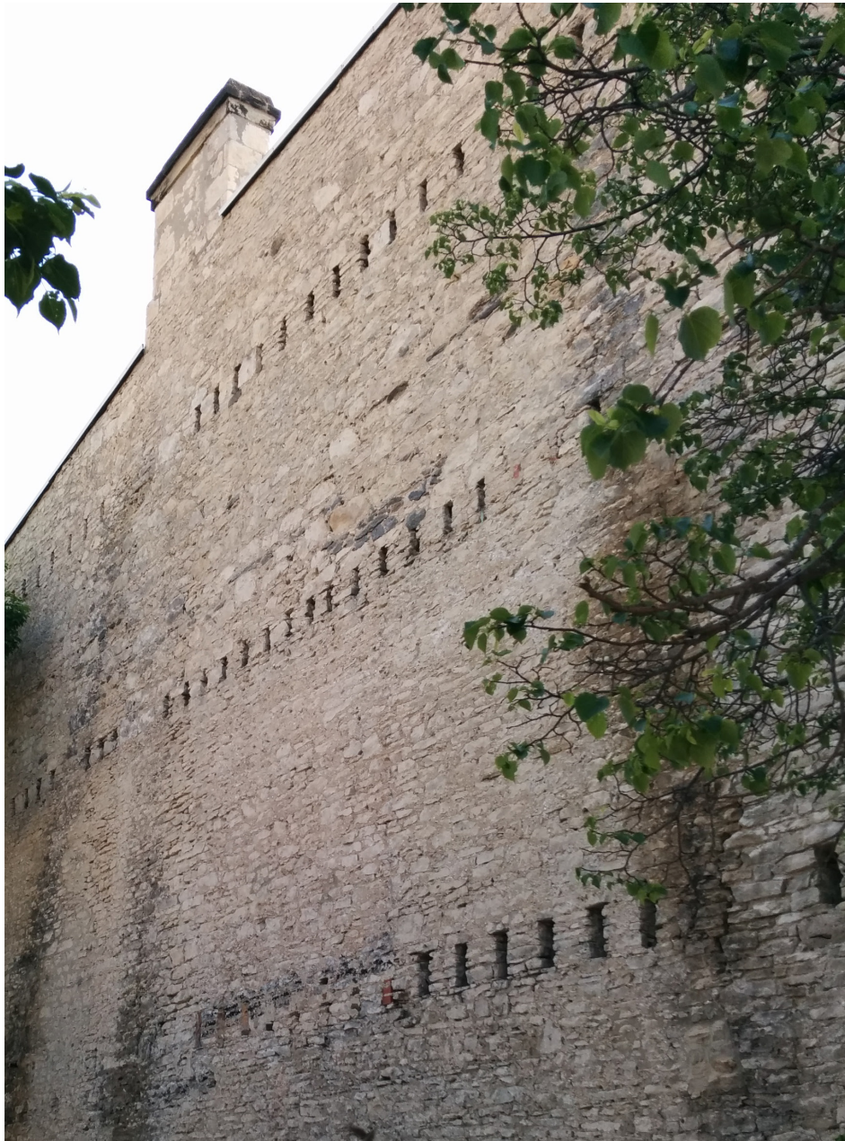
Fig. 2.6. Remaining masonry party wall inhabited by sparrows.
