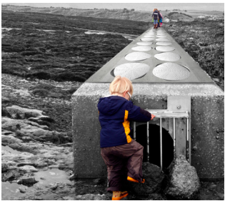
Fig. 1.9. Urchin Tile designed by Daniel Metcalfe for an outfall pipe in Hannafore beach.
