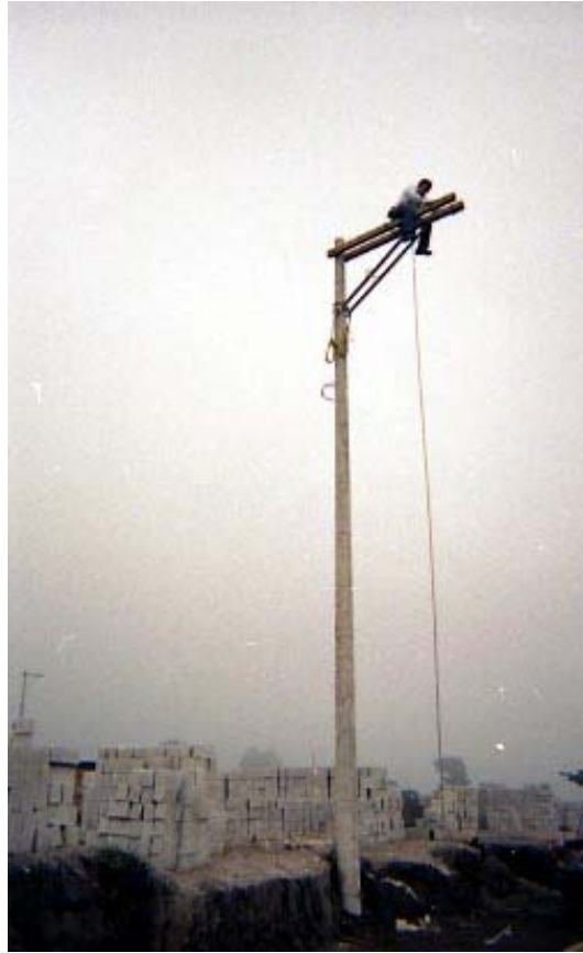
Figure 5.13 Bringing electricity to Totolyá (photographed by Antonio)
