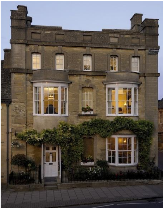
Figure 19. Hope House, Woodstock, Oxfordshire (1720) 209
