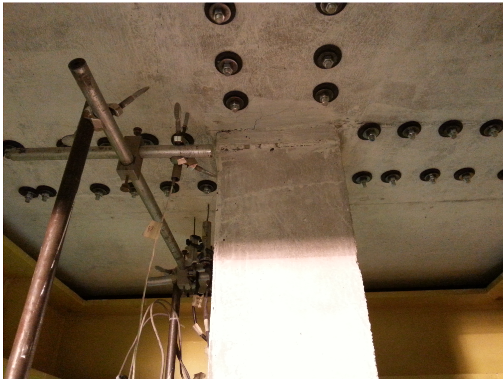
(b) Cracks at 2% drift
